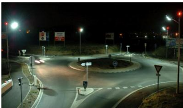
Figure 2 The roundabout lighting LED system
