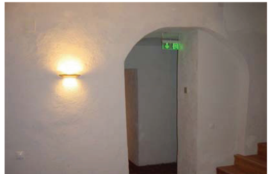
Figure 1 Lighting of the basement entry, Building A, Black Eagle
