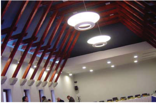
Figure 3 Lighting of the rebuilt conference room, Building C, Black Eagle
