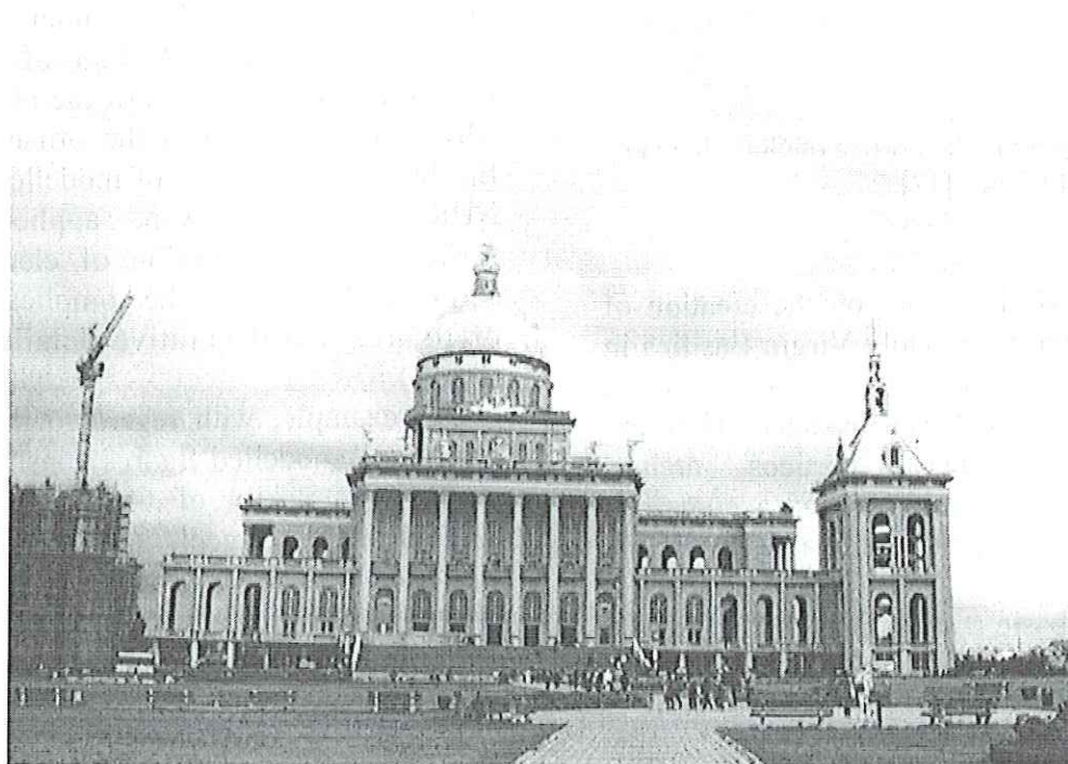
Figure 1 The front facade of the Basilica of Licheń [12]
